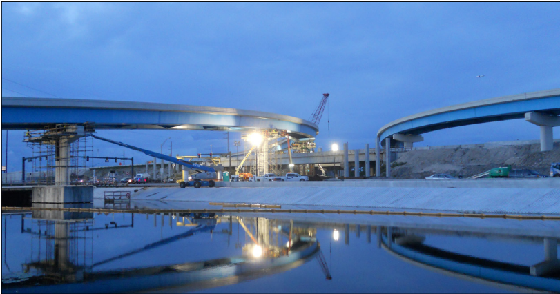
Construction of I-595; completed in 2014
